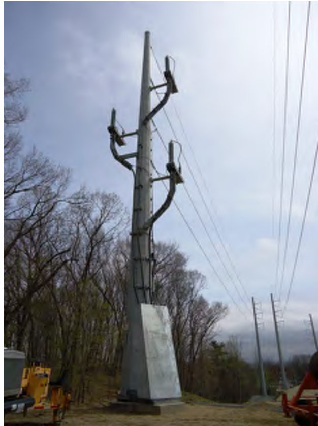
Figure 4-6: Typical 161kV Transition Structure
