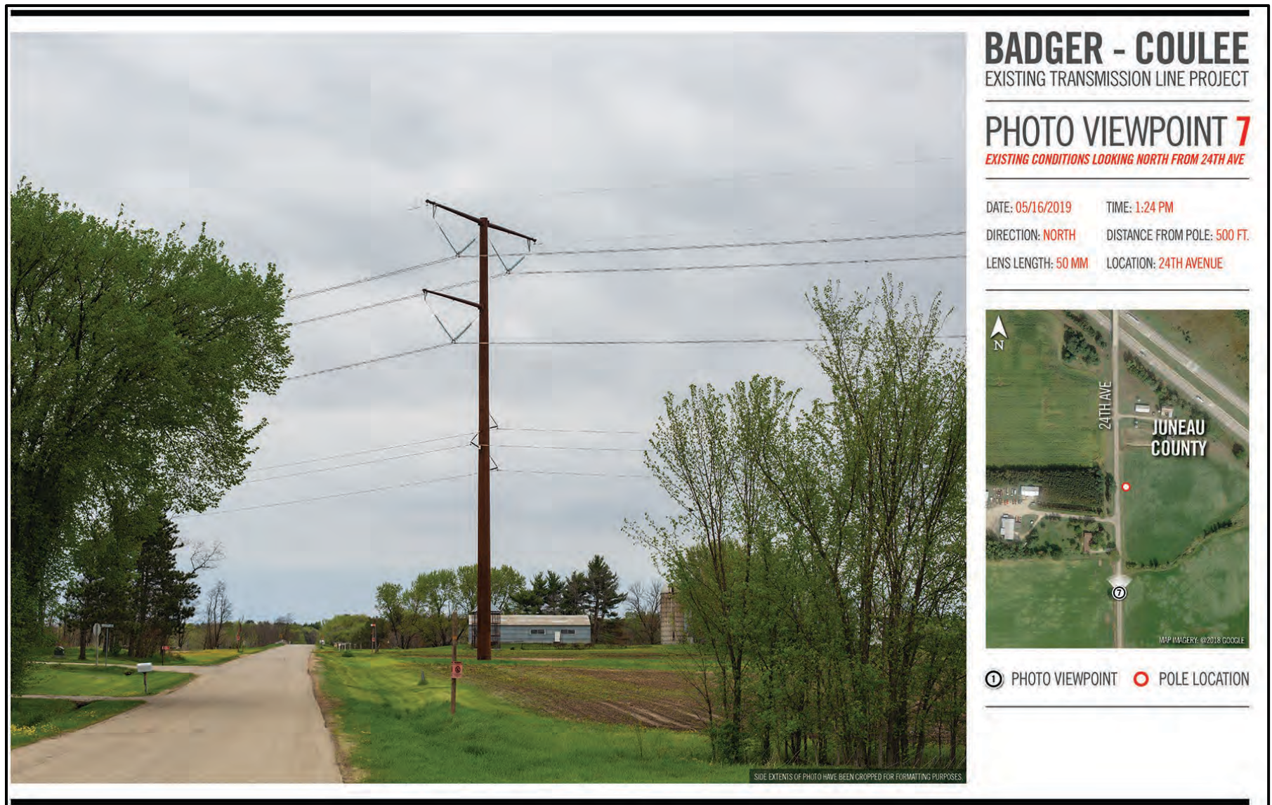
Figure 3.11-9. Representative photograph from Photo Viewpoint 7 within 500 feet of the Badger-Coulee Transmission Line project.
