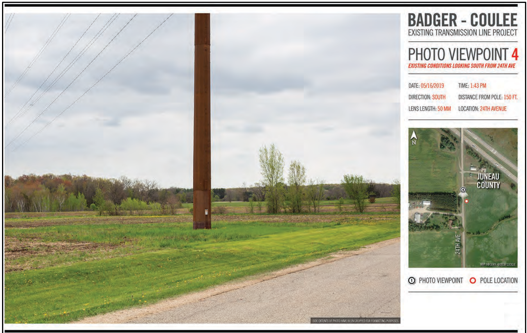
Figure 3.11-6. Representative photograph from Photo Viewpoint 4 within 150 feet of the Badger-Coulee Transmission Line project.
