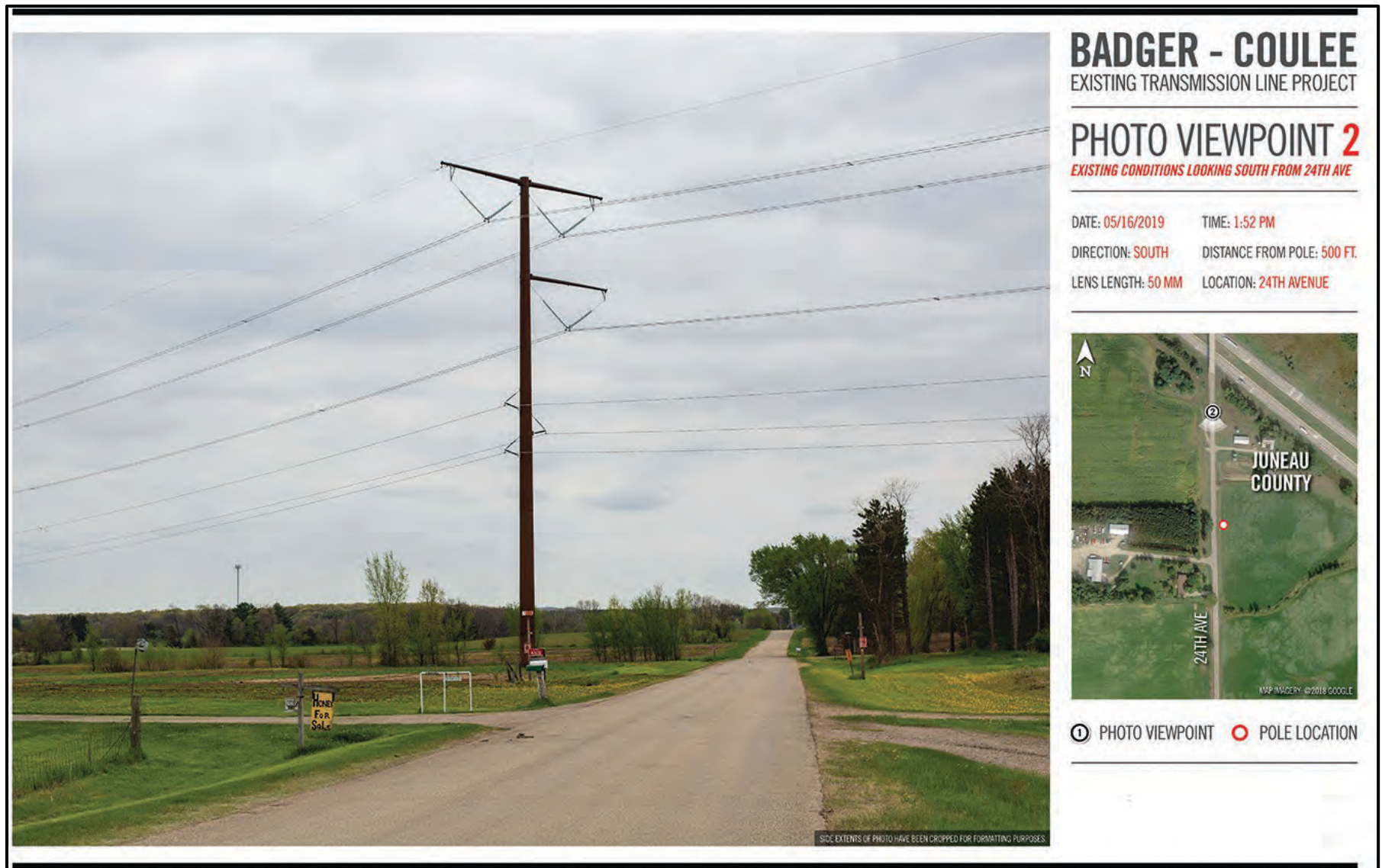
Figure 3.11-4. Representative photograph from Photo Viewpoint 2 within 500 feet of the Badger-Coulee Transmission Line project.
