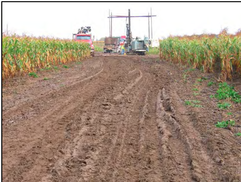
Figure D-1. Rutting of topsoil in cropland—no soil mixing.
