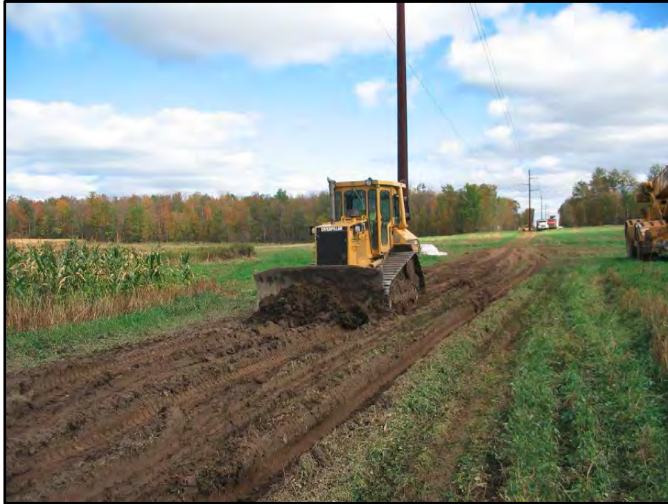
Figure D-2. Ruts being smoothed with blade.
