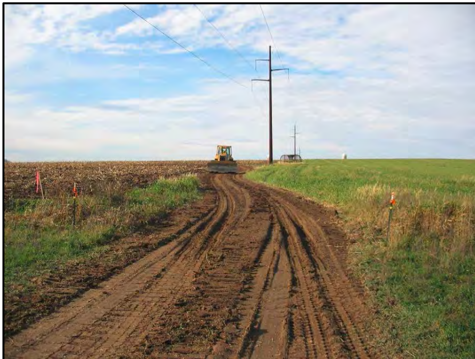
Figure D-3. Smoothing out ruts by backblading with a dozer.
