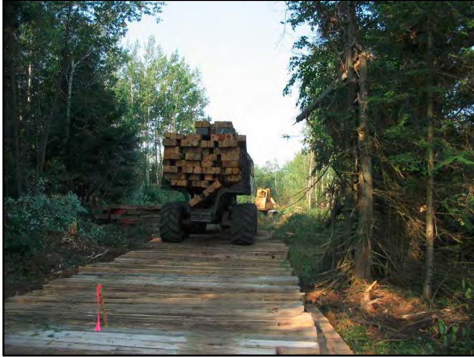
Figure D-7. Timber mats being placed in wooded wetland.
