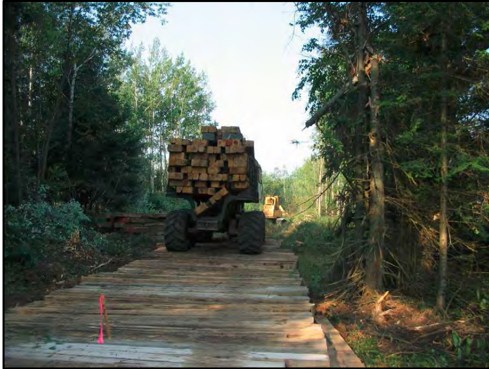
Figure 2.4-8. Timber mats being placed in wooded wetland.
