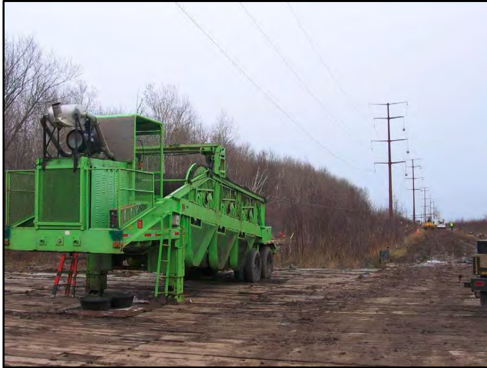
Figure 2.4-14. Pulling the conductor through the structure arms.
